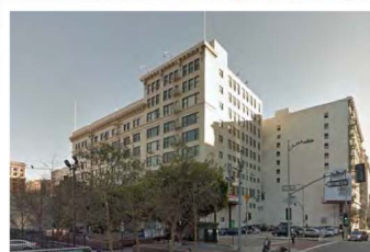
Junipero Serra Office Building
